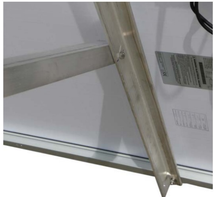
Attach leg to panel kit.
